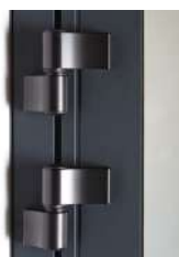
Paumelles et joint anti-pince doigts
